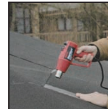
Weld Roofing Felt
